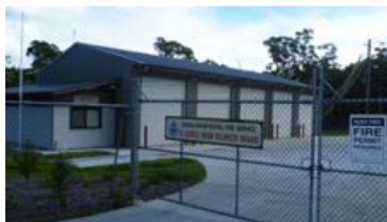
RFS base with new pole in background
