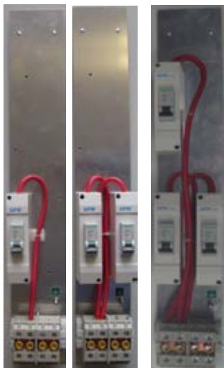
B0031, B0032, B0033 PWC Street light Switch Packs
