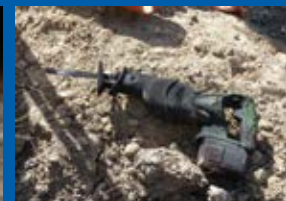
Reciprocating saw used to cut ducts
