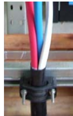
LV 4c 240mm 2 Al cable fixed to LV frame
