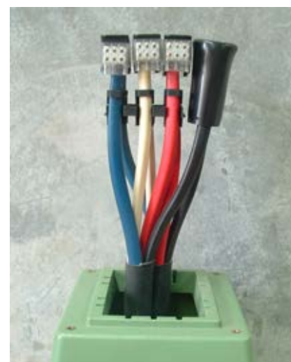
Left is a picture showing the shearbolt 2 mains termination for 240mm 2 4c stranded or solid Aluminium cable, approved for the Integral Energy and Energy Australia networks.
